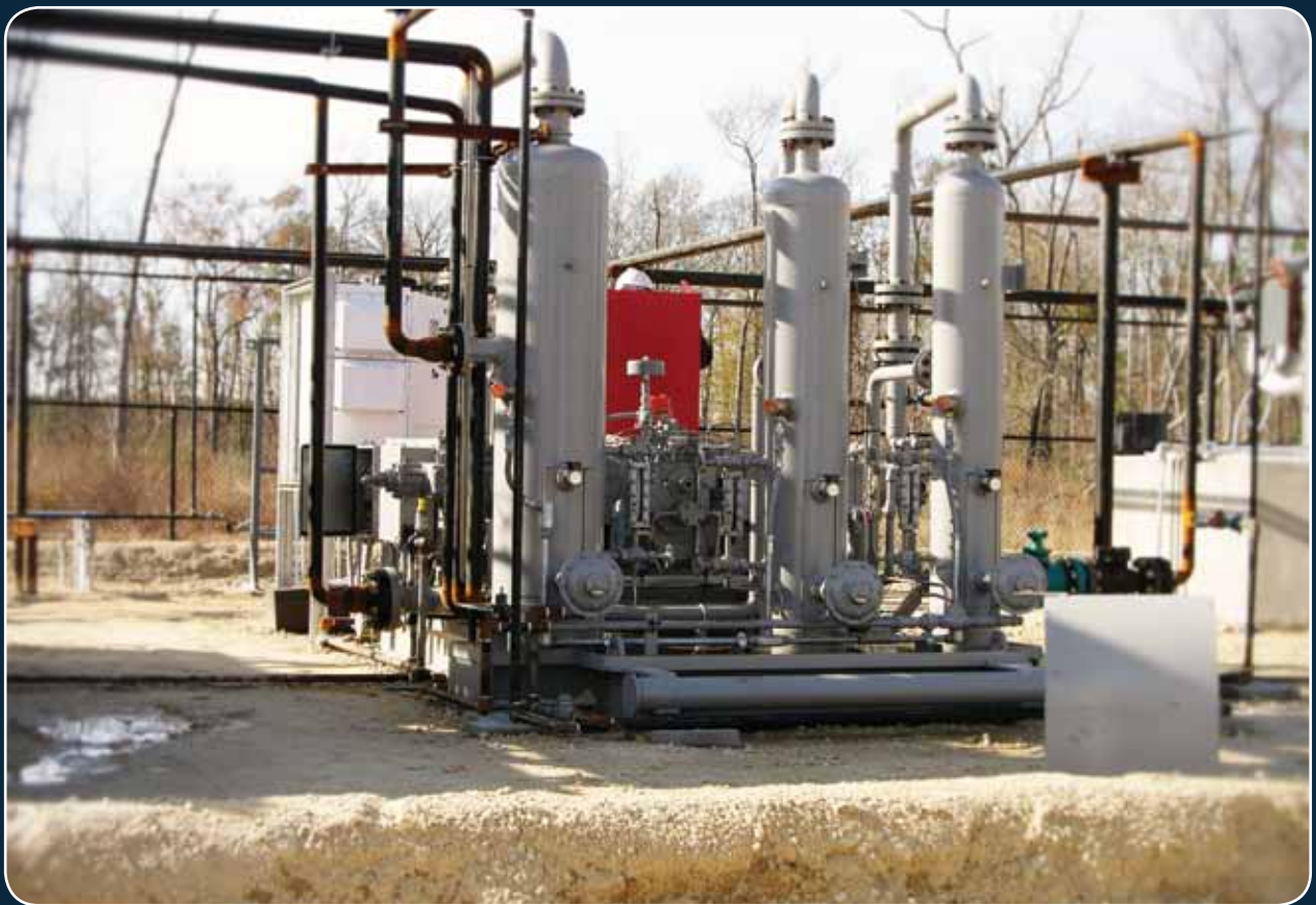
Engineered Concepts packaged this electric compressor as part of an emission free well pad.
