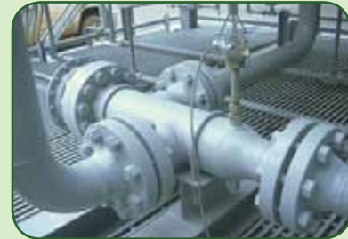
Engineered Concepts PICT technologies address air cooled compressor problems (out of control recycles) during cold weather operation.
